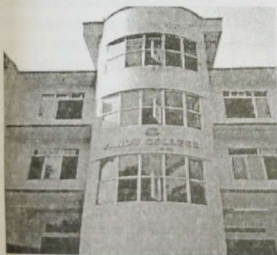
Fig. 1.8. Old Building (Source: Internet)
