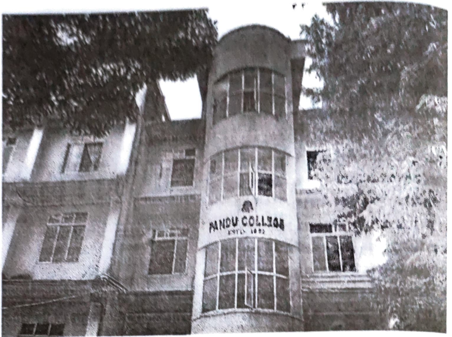
Administrative Building, Pandu College
